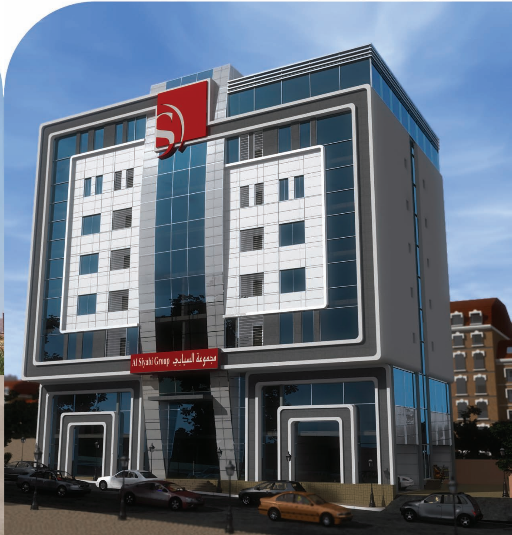
Al Seyabi Group Headquarters - Commercial cum Residential building at B.C.C Bousher (Ongoing)
