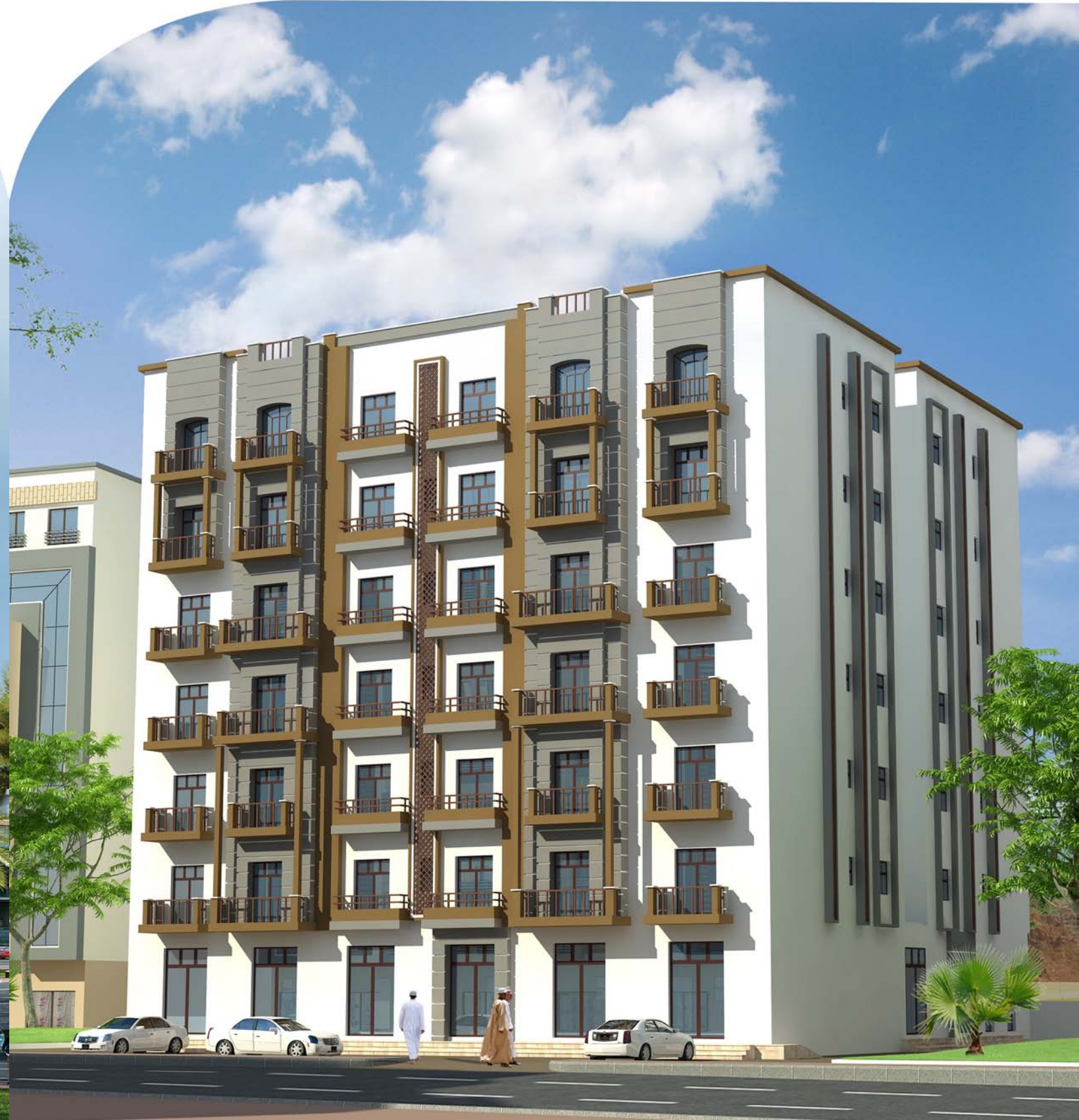
Commercial cum residential building at Bousher, opp. Bousher Dunes (Ongoing)
