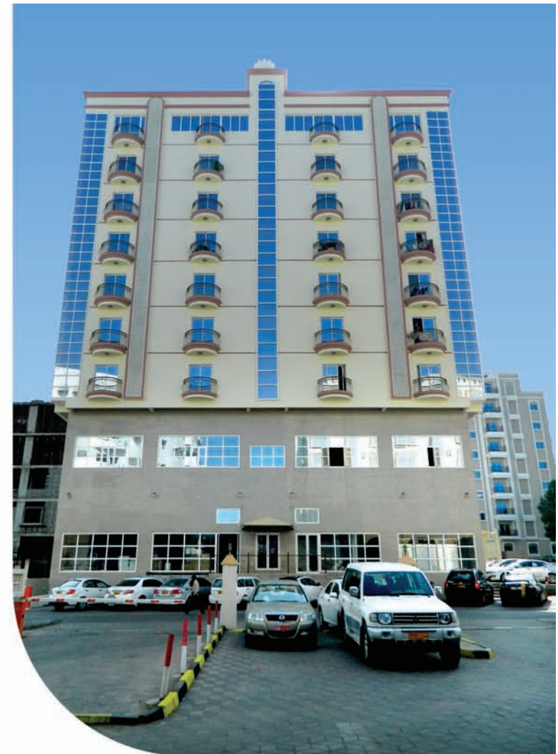
Commercial cum Residential building in al-Khuwair (behind Mustafa Sultan enterprises)
